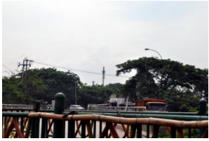
Tower at natural gas refinery near Jakarta, Indonesia
